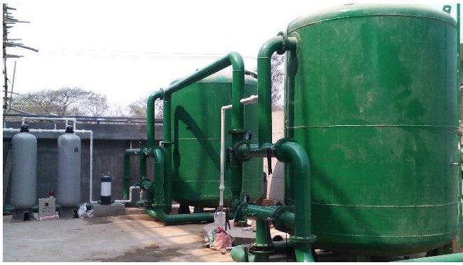
Pre-treatment, Water Softener, Micron Filter, UV System, Columbia Washing Plant Ltd.
