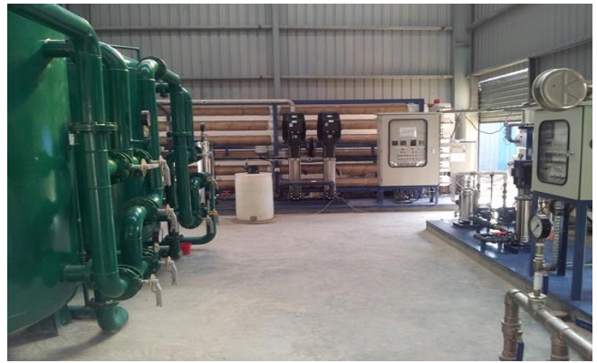
Pre-treatment, RO System, Mixed Bed System, Baraka Patenga Power Ltd.
