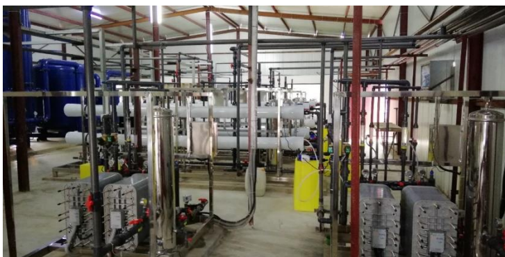
Pre-treatment, Water Softener, RO System, EDI System, Oxidation Chamber, United Mymensingh Power Ltd.
