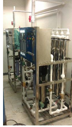
Pre-treatment, Water Softener, Oxidation Chamber, RO System, UV System, Square Hospitals Ltd.
