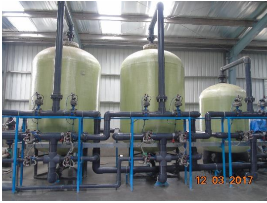
Pre-treatment, Water Softener, ACI Healthcare Ltd.
