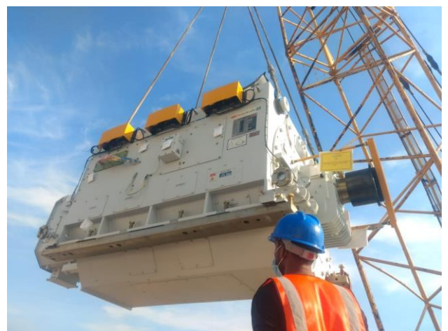
Turbine, Alternator, Condensor Erection work, Orion Power Sonargaon Limited
