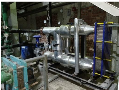
03 Nos. 15 m 3 /h @65°C, Heat Recovery Hot Water system from Engine Jacket Water at Montex Fabrics Ltd, Nayapara, Kashimpur, Gazipur.
