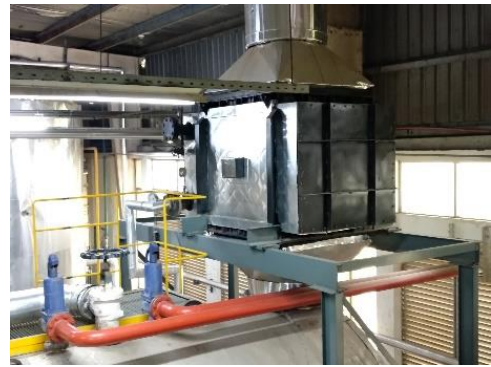
5 Ton, 6 Ton, 7 Ton (two) Economiser installed at Envoy Textile, Jamirdia, Bhaluka, Mymensingh
