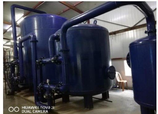
Pre-treatment, Water Softener, RO System, EDI System, Oxidation Chamber, United Mymensingh Power Ltd.
