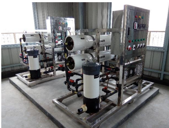
Pre-treatment, Water Softener, RO System, Asgar Ali Hospital
