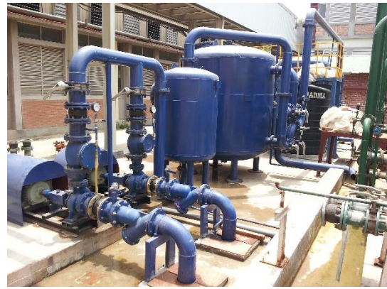
Pre-treatment, Water Softener, Oxidation Chamber, Envoy Textiles Ltd.
