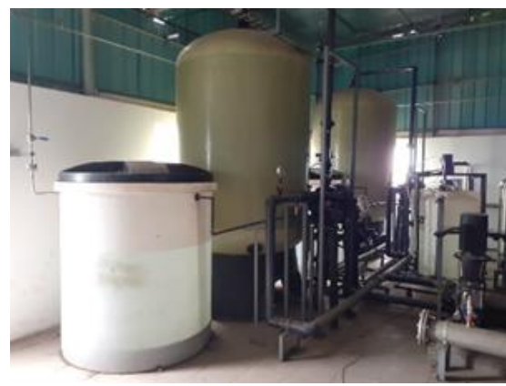
Pre-treatment, Water Softener, Beximco Pharmaceuticals (Unit-III) Ltd.
