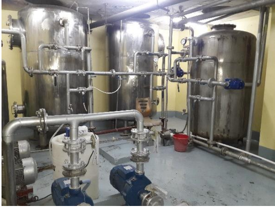
Pre-treatment, Water Softener, Oxidation Chamber, RO System, UV System, Square Hospitals Ltd.
