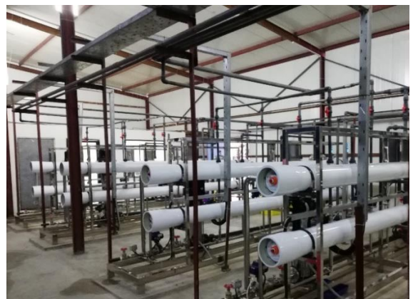
Pre-treatment, Water Softener, RO System, EDI System, Orion Power Rupsha Ltd.
