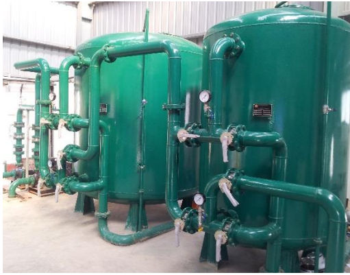
Pre-treatment, RO System, Mixed Bed System, Baraka Patenga Power Ltd.
