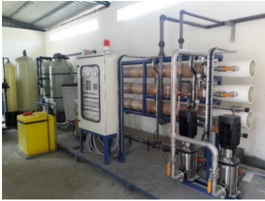
Pre-treatment, Water Softener, RO System, EDI System, Oxidation Chamber, Dhaka Southern Power Generation
