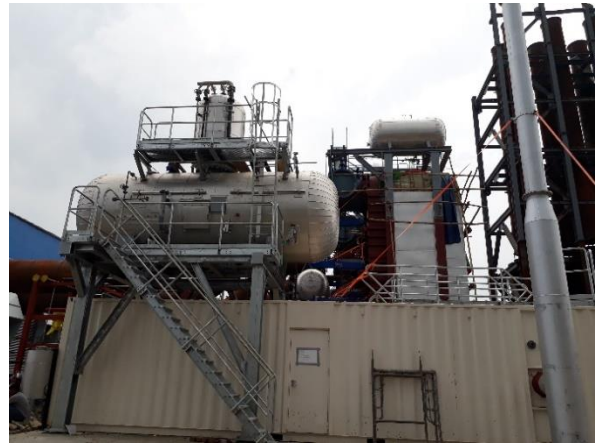
Aux. Boiler Erection Works, Orion Power
