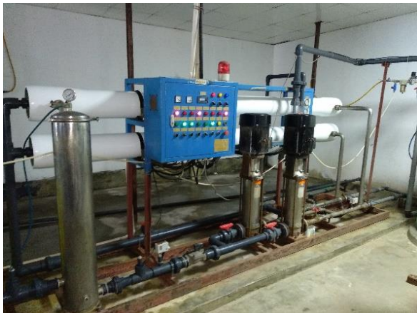
Pre-treatment, Water Softener, RO System, EDI System, UV System, Square Toiletries Ltd.
