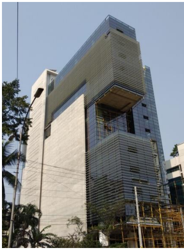
BTI Landmark, Gulshan Avenue (STP & WTP)
