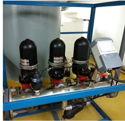
Raw water & Treated water Delivery Pump & Disc filter (Rain water Treatment plant) Saiham Tower
