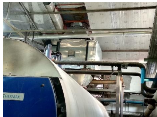
Economiser installed at Montex Fabrics Ltd. Nayapara, Kashimpur, Gazipur, Dhaka
