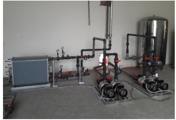
Pre-treatment, Water Softener, RO System, EDI System, Oxidation Chamber, Dhaka Southern Power Generation
