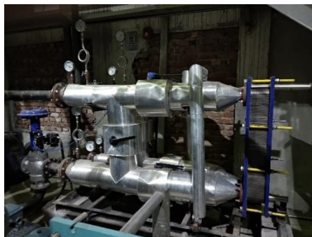
03 Nos. 15 m 3 /h @65°C, Heat Recovery Hot Water system from Engine Jacket Water at Montex Fabrics Ltd, Nayapara, Kashimpur, Gazipur.
