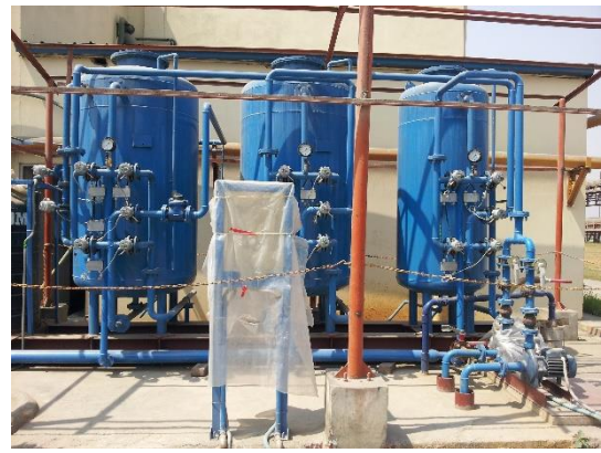
Pre-treatment, Water Softener, Oxidation Chamber, Envoy Textiles Ltd.
