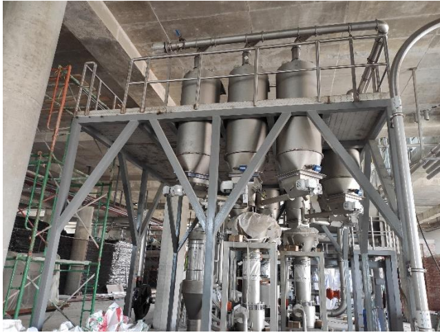
Erection Work at Akij Bakers Ltd
