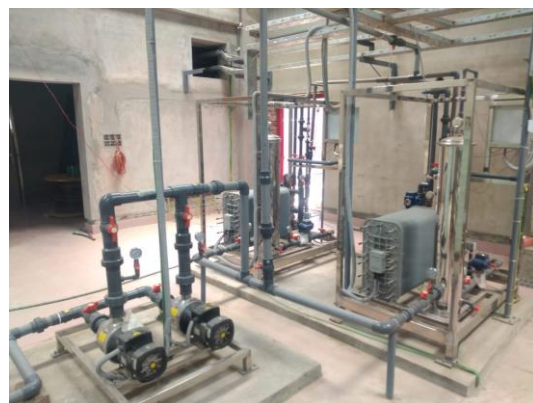
Pre-treatment, Water Softener, RO System, EDI System, Orion Power Sonargaon Ltd.
