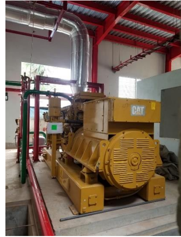
Generator Erection Work at American & Efid Ltd.
