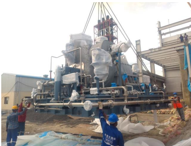
Turbine, Alternator, Condensor Erection work, Orion Power Sonargaon Limited
