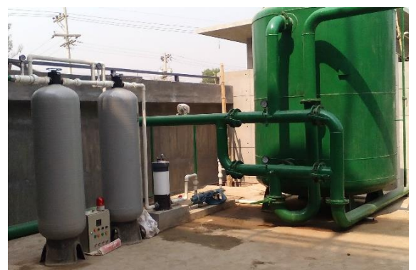
Pre-treatment, Water Softener, Micron Filter, UV System, Columbia Washing Plant Ltd.
