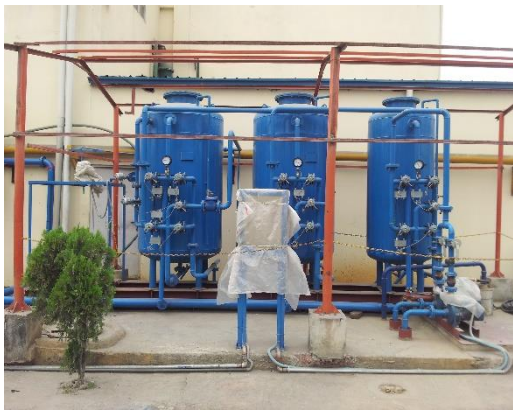
Pre-treatment, Water Softener, CEMEX Cement (BD) Ltd.
