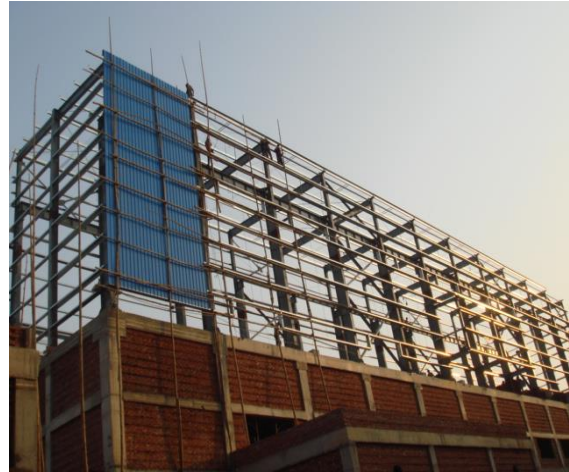
Pre-Fab Steel Building, Knittex Dresses
