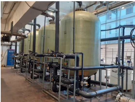
Pre-treatment, Water Softener, Beximco Pharmaceuticals (Unit-III) Ltd.
