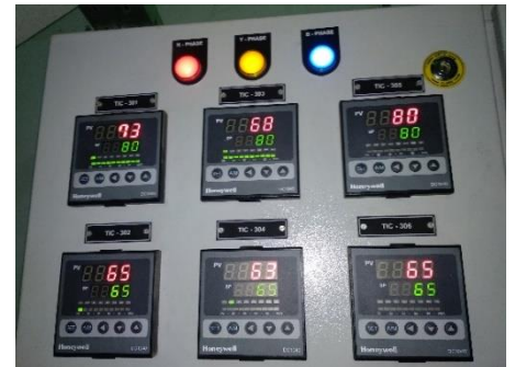
03 Nos. 15 m 3 /h @65°C, Heat Recovery Hot Water system from Engine Jacket Water at Montex Fabrics Ltd, Nayapara, Kashimpur, Gazipur.
