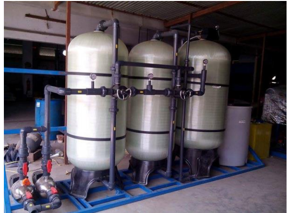
Pre-treatment, Water Softener, RO System, EDI System, UV System, Square Toiletries Ltd.
