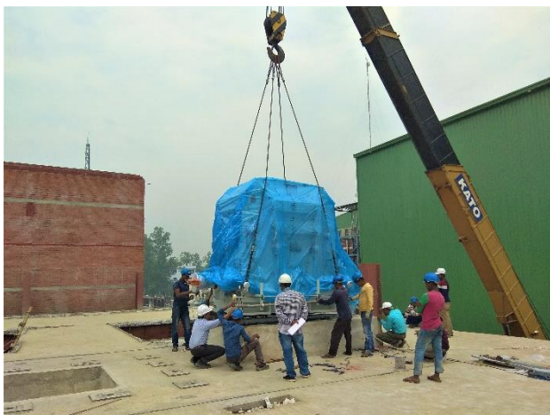
Confidence Power Bogra Limited (Installation of Equipment)
