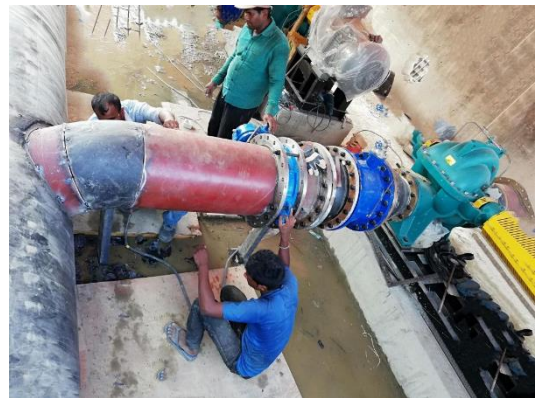
Cooling System Erection work, UMPL
