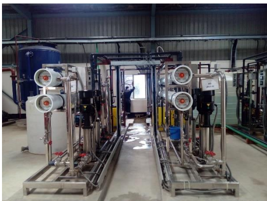
Pre-treatment, Water Softener, RO System, EDI System, Confidence Power Rangpur Ltd.
