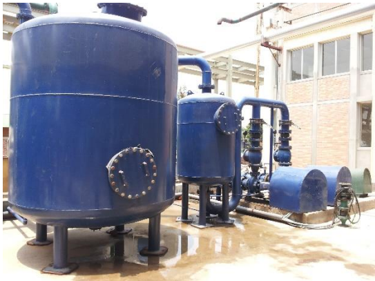
Pre-treatment, Water Softener, Oxidation Chamber, Envoy Textiles Ltd.
