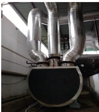
1 waste heat recovery saturated steam boiler at Chaity Knit Composite Ltd, Sonargaon, Narayanganj (3 Gas engine waste heat connected to a common EGB)
