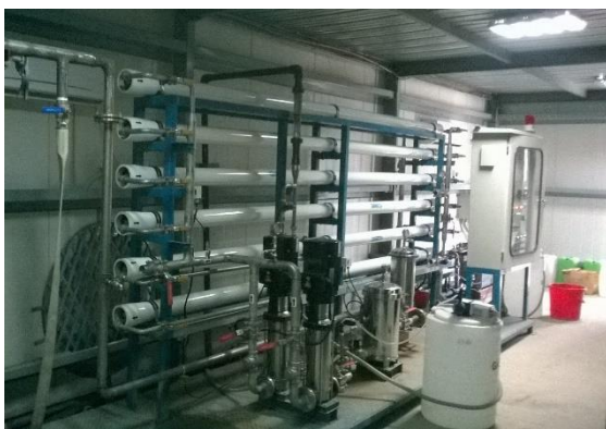
Pre-treatment, Water Softener, RO System, EDI System, Orion Power Sonargaon Ltd.
