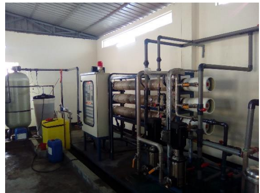
Pre-treatment, Water Softener, RO System, EDI System, Oxidation Chamber, Dhaka Northern Power Generation
