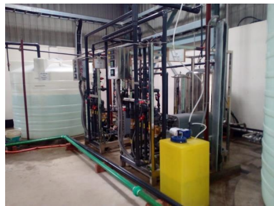
Pre-treatment, Water Softener, RO System, EDI System, Confidence Power Rangpur Ltd.
