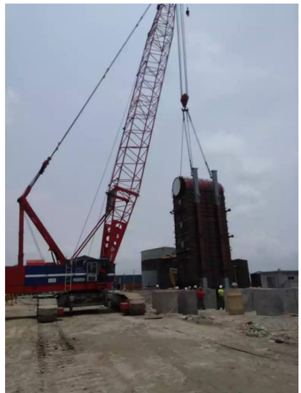
EGB Boiler installation work, OPRL
