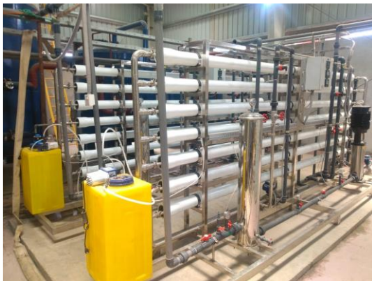
Pre-treatment, Water Softener, RO System, EDI System, Orion Power Sonargaon Ltd.
