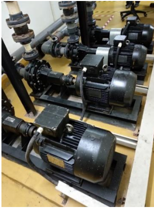
Raw water & Treated water Delivery Pump & Disc filter (Rain water Treatment plant) Saiham Tower
