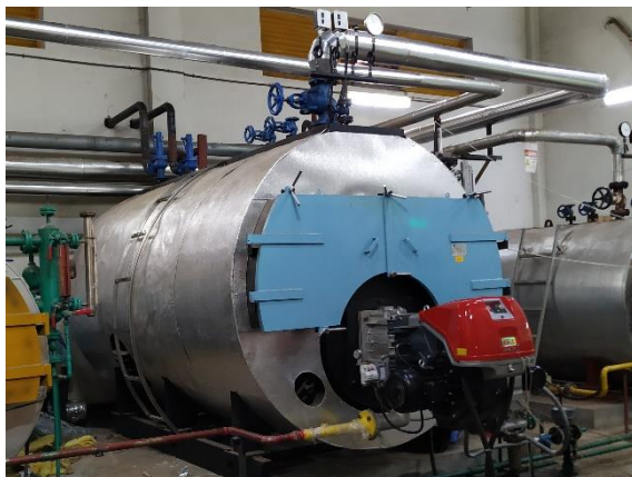
4TPH Steam Boiler, Towa Personal Protective Device
