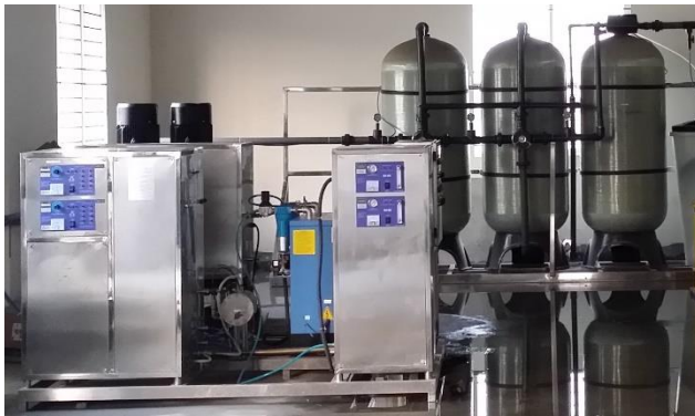
Pre-treatment, Water Softener, RO System, EDI System, Oxidation Chamber, Dhaka Northern Power Generation
