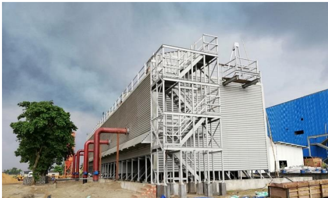
Cooling Tower Erection work, UMPL
